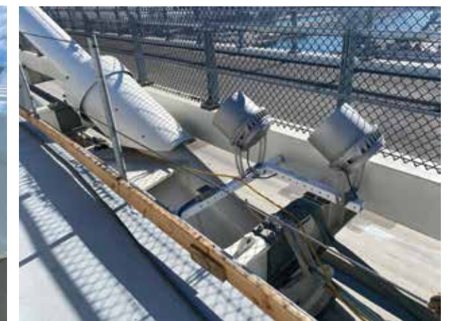
LED lights are mounted to illuminate the cable-stays and towers.
